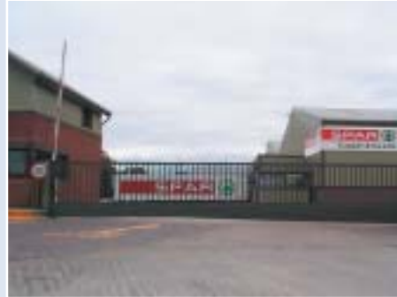
LoTracker sliding gate with skirt to accommodate the slope on this particular site.
